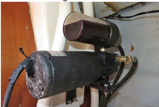
No leaks at hydraulic power pack
