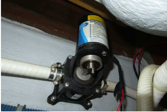
Shower drain pump without leak
