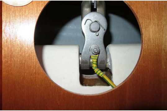
No damages at shroud tie rod attachments
