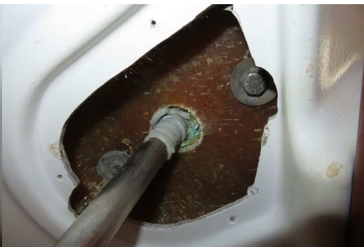
No cracks below shroud deck plates
