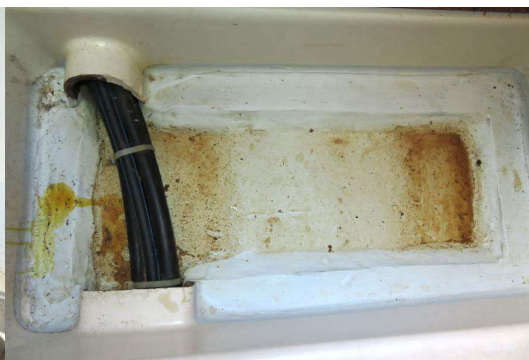
No cracks at interface of liner and hull
