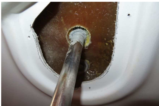
No cracks below shroud deck plates
