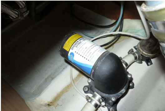
Refrigerator drain pump without leak
