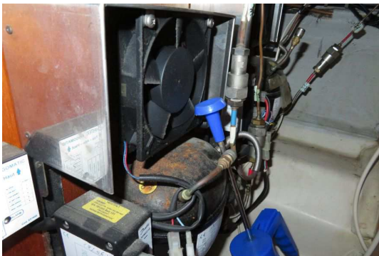
Compressors minor corrosion
