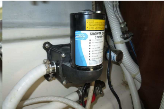
Shower drain pump without leak
