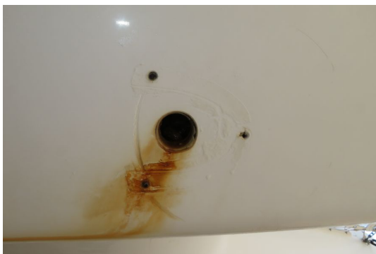
Clamshell drain cover missing at bridge deck underside
