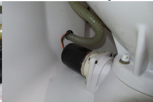
No leaks at toilet discharge pump
