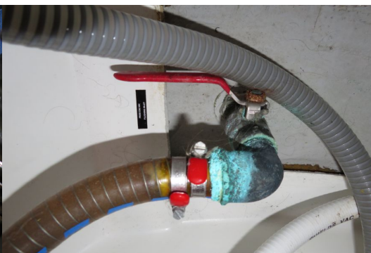
Small leak at owner toilet inlet valve
