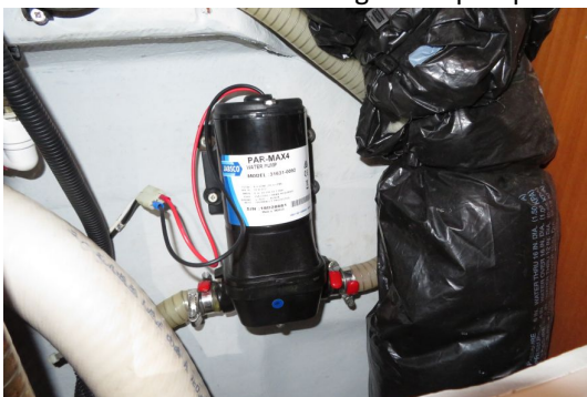
No leaks at toilet flushing water pump
