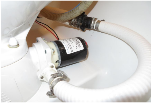
No leaks at toilet discharge pump
