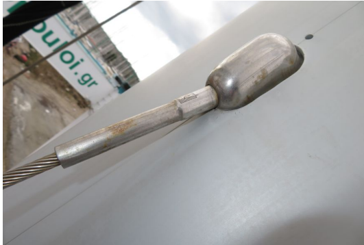
Intermediate upper swages without broken wire
