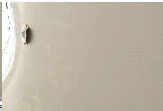
Crazing at bridge deck underside
