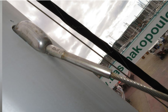
Intermediate upper swages without broken wire
