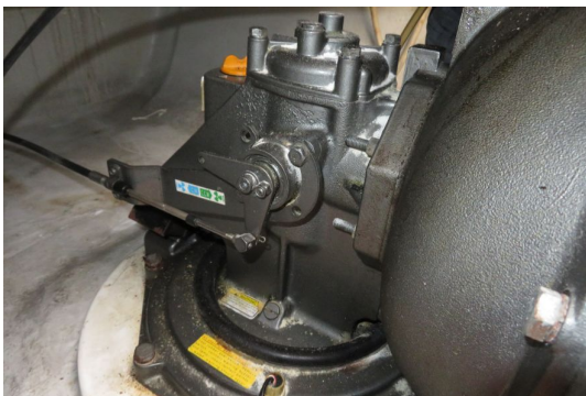
No leaks at seal
