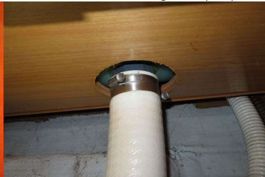
No leaks at owners holding tank
