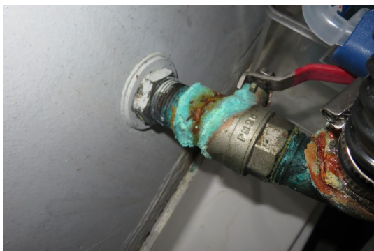
Small leak at sink drain valve
