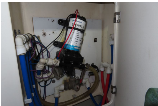
Fresh water pump no leaks
