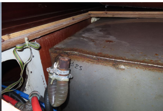
Stainless tank no sign of leaks
