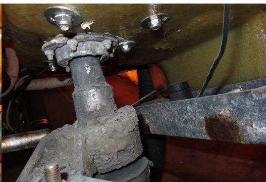
Leaks from deck level leading to corrosion
