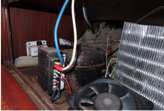
Refrigerator compressor requires repaint
