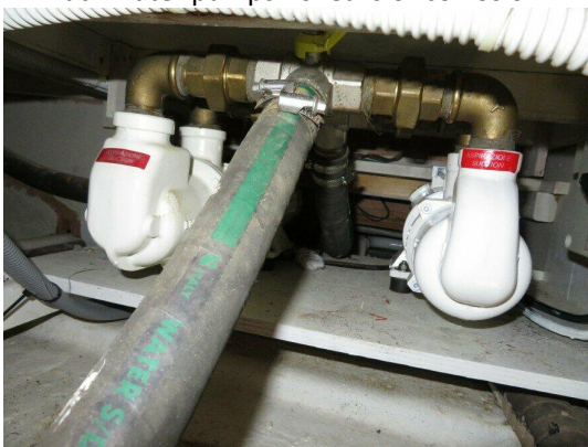
Black grey water pumps no leaks or corrosion
