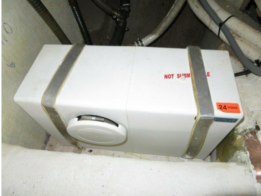
Grey water sumps externally intact and secure
