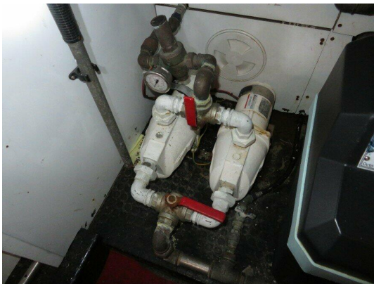
Black water pumps no leaks or corrosion
