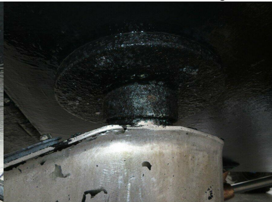
No corrosion at bearing
