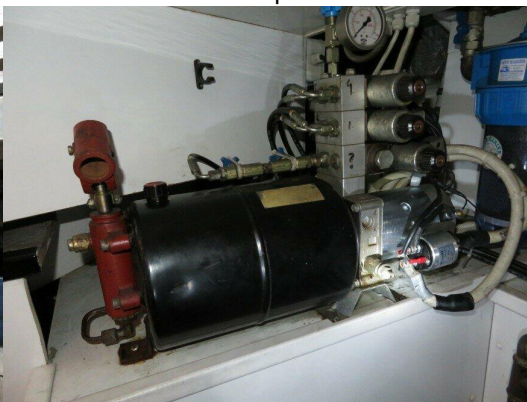
Hydraulic power pack without leaks or corrosion
