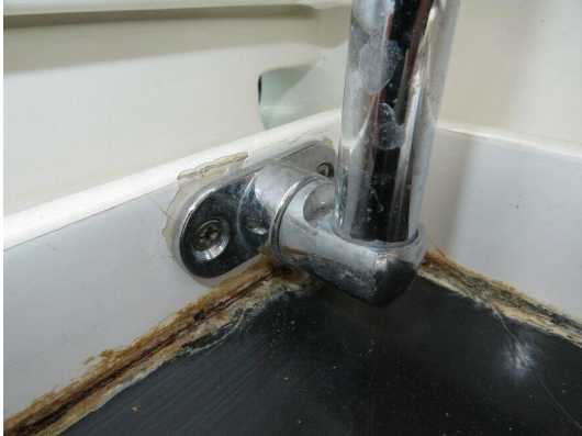
Holding up strut for wet bar to rescrew
