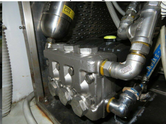
New watermaker high pressure pump
