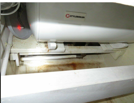
Water heater no corrosion or leaks
