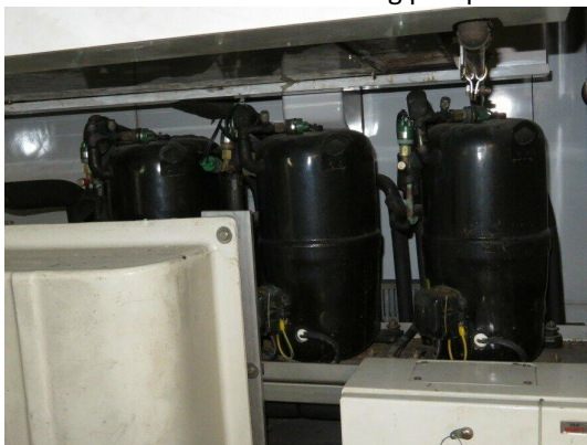
Compressors with coatings intact
