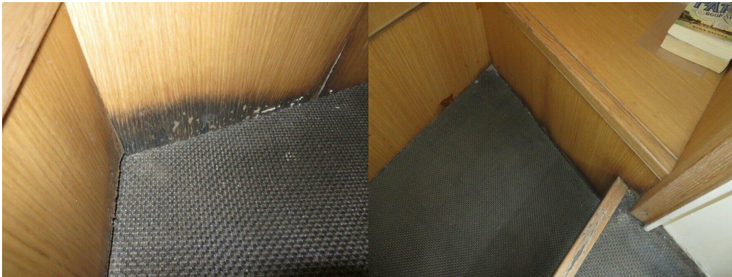
Crew accommodation some blackening to panelling at floor level
