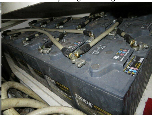
Batteries bulging
