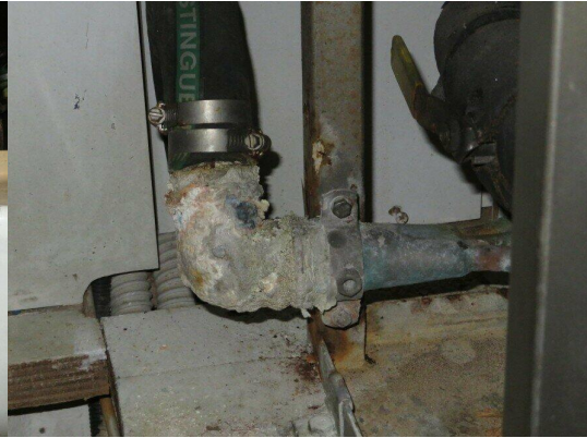
Minor previous leak seawater elbow
