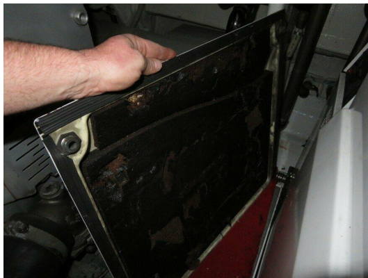
Generator soundproofing to renew
