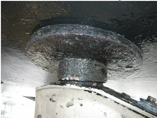
No corrosion at bearing
